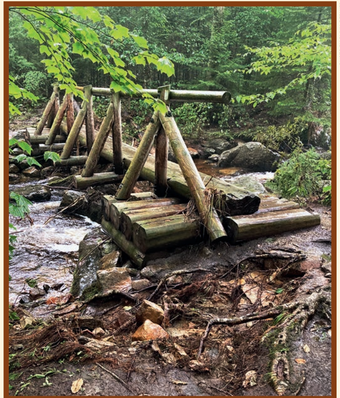
Homer Stone Brook Bridge, shown here after the 2023 flood, will be replaced with a glulam stringer bridge.
