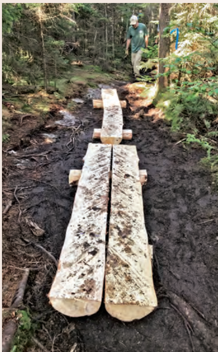
Your membership dues at work: native puncheon installed on Laraway Mountain.
