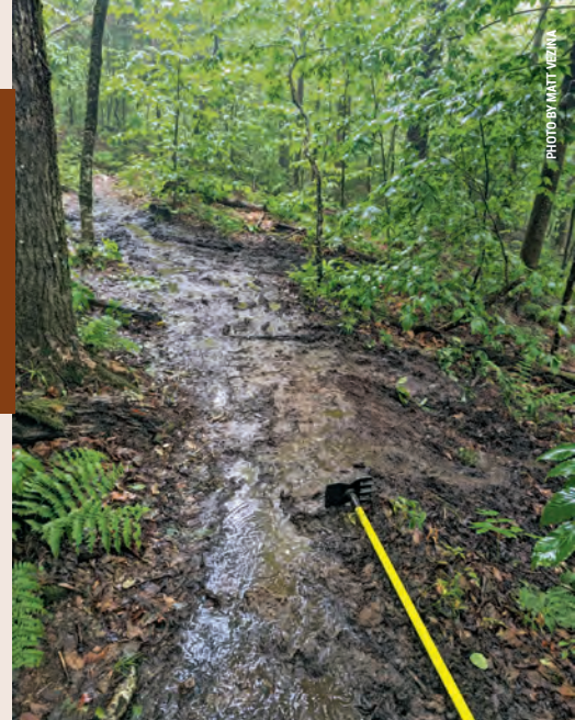
Deberming, or removing the raised edge of a mudpit with a hoe (or your foot!) so that water can drain, is the first step to alleviating mud.
