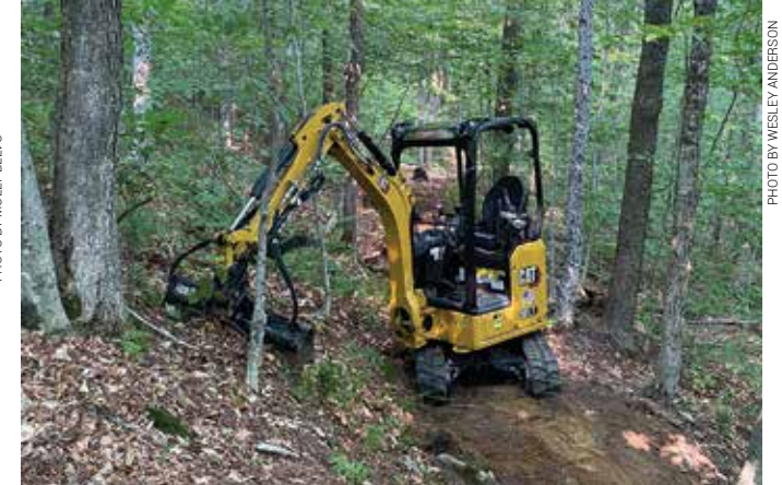
GMC used a mini excavator to cut new tread on Belvidere Mountain.
