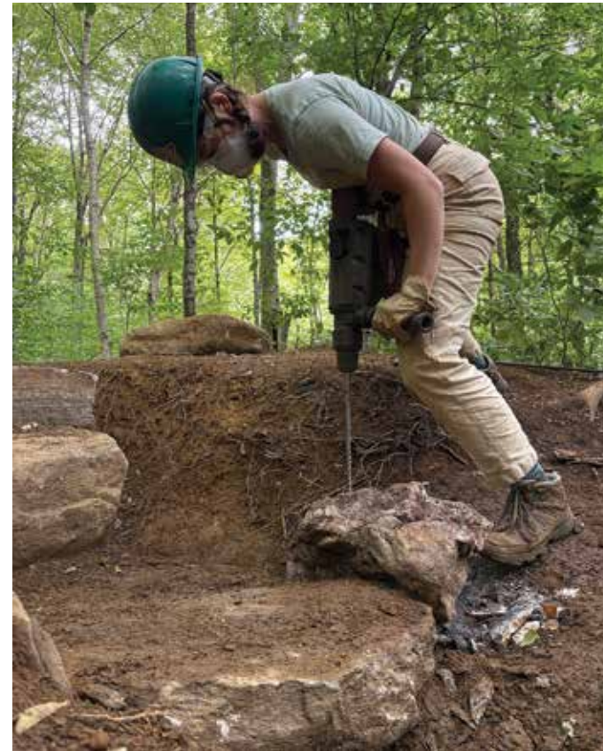
Pinning a rock in place on the new LT route on Belvidere.
