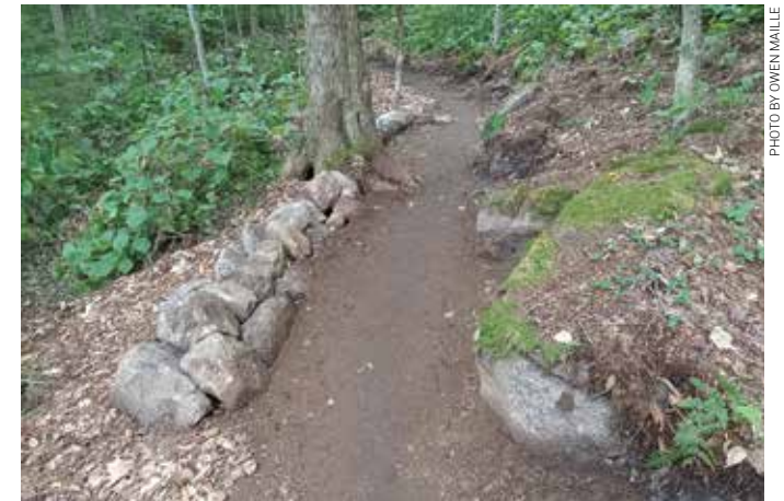
New turnpike on a short relocation on the LT/AT south of Risky Ranch Road.
