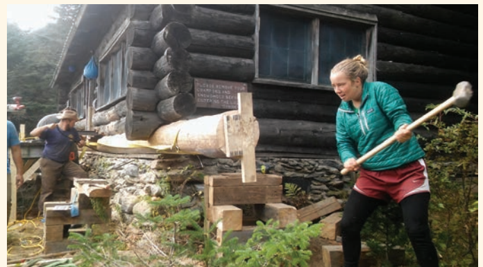
2016 Taft Restoration—crew member Daley whacks a replacement log into place.
