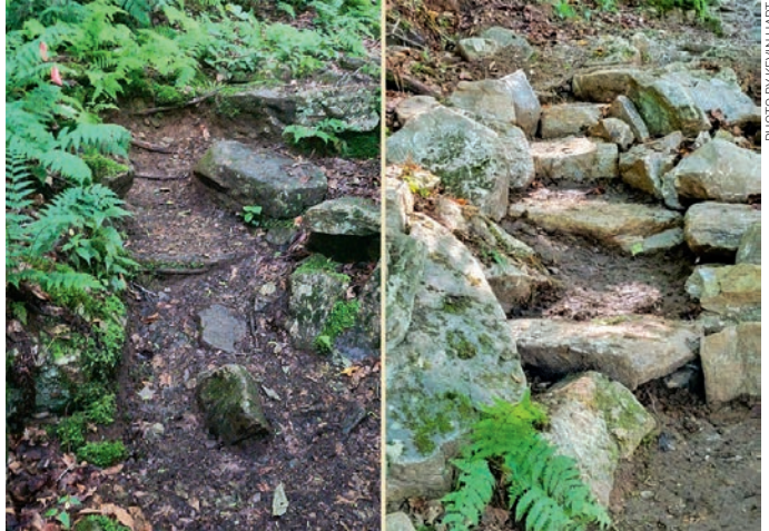
Crews replaced an eroded gully with stone steps on the LT/AT near Route 9.
