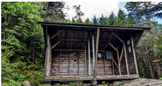
Puffer Shelter, first built in 1975. GMC Construction Crew reset the piers and added interior stabilization.
