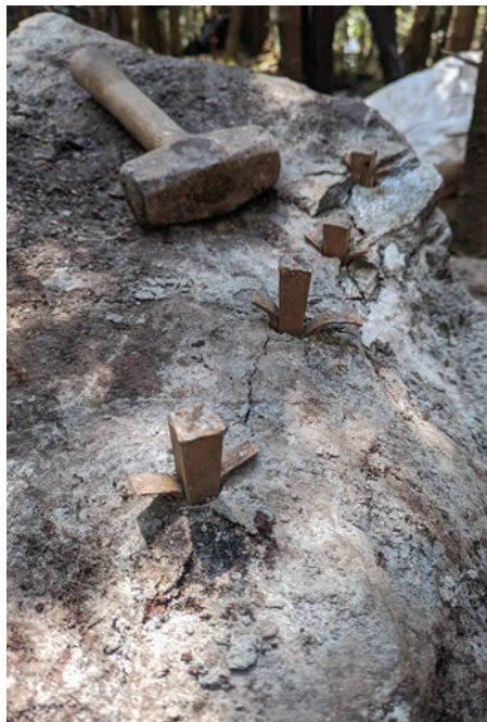
Installing rebar to set stone steps on Burrows Trail.
