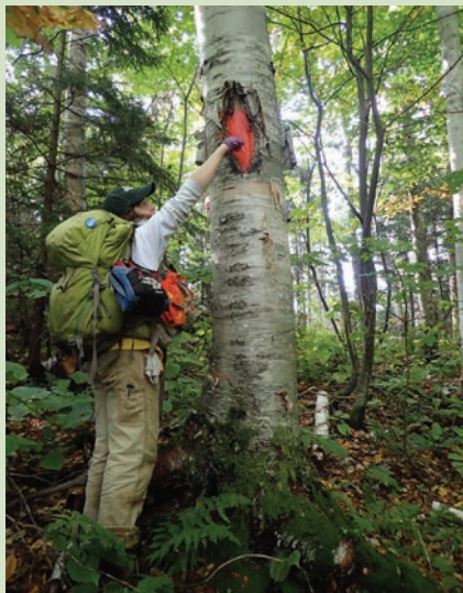
A well-marked boundary line includes painted blazes on trees, a rebar pin at each corner, and signage indicating the owner.
