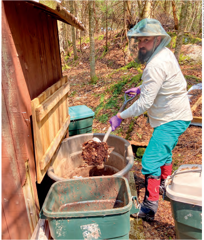
Caretaker Lead Dan Lane stirs a composting privy run at Montclair Glen during training.
