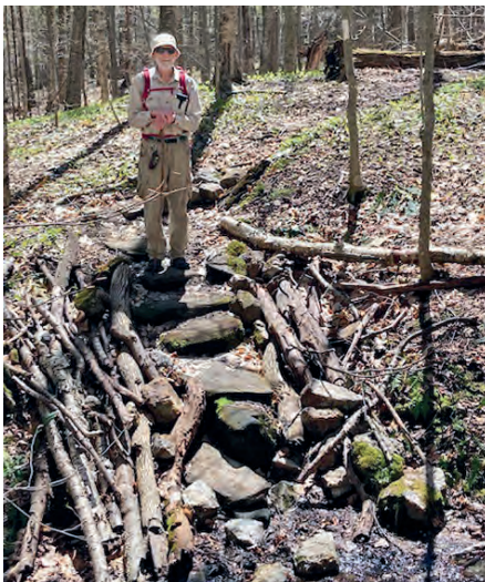
Dick Andrews at log-and-rock-filled staircase gullies on the AT north of Thistle Hill Shelter.
