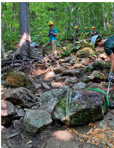
Clara guides a rock over obstacles with a rockbar while Andrew operates the Griphoist.
