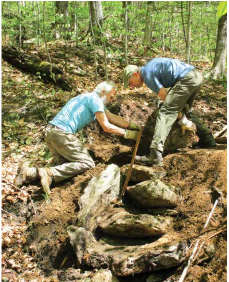
MONTPELIER SECTION: Building stone steps on Long Trail
