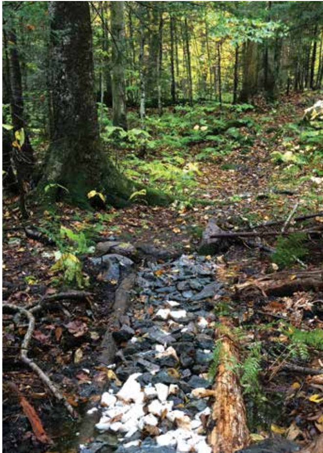
STERLING SECTION: New turnpike built by Sterling Section members on the Chilcoat Trail
