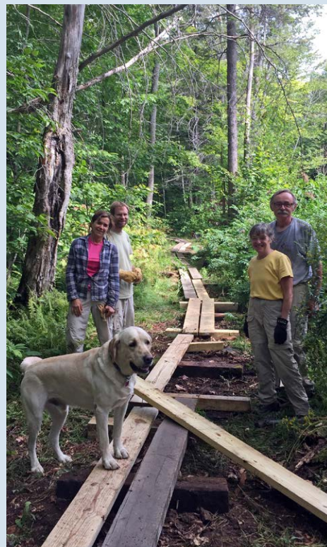
Manchester Section puncheon replacement on the Long Trail north of the Bromley Brook crossing
